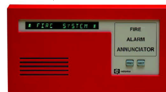
Fire Command Center and Fire Annunciator
